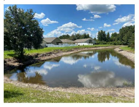
Photo of Pond bank erosion below the high water line.
